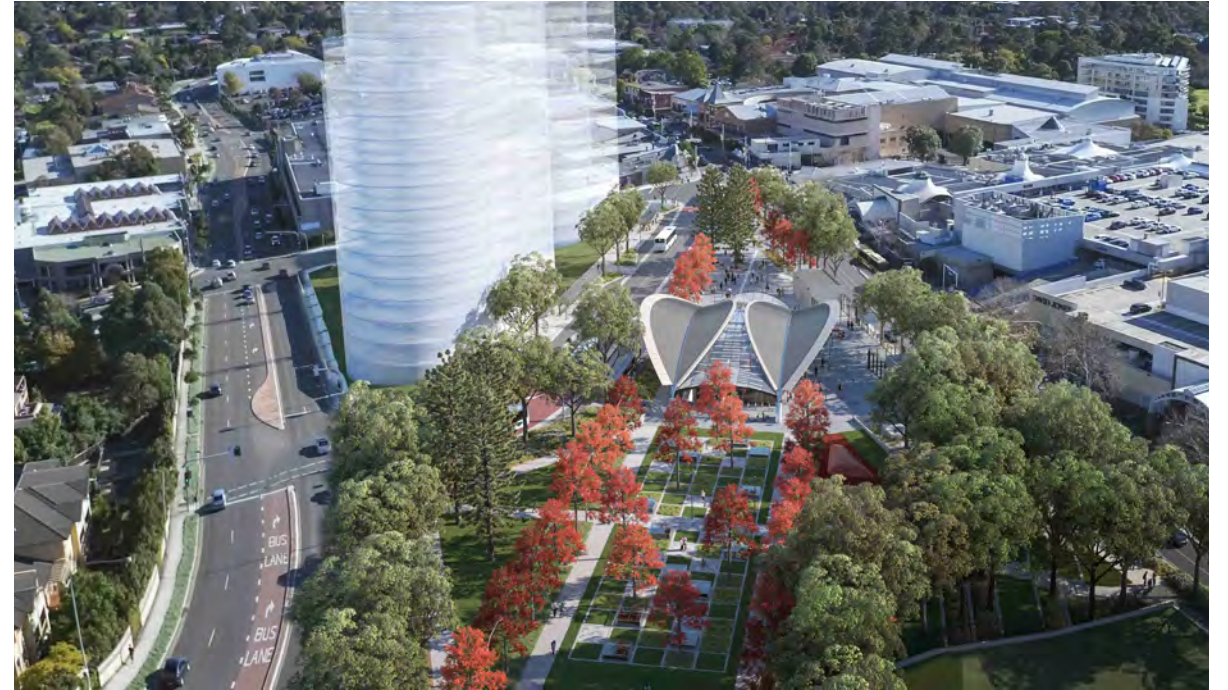
Castle Hill Station - the order of the station grid & grove, framed by native trees, set within the complexity of contemporary urban development.
